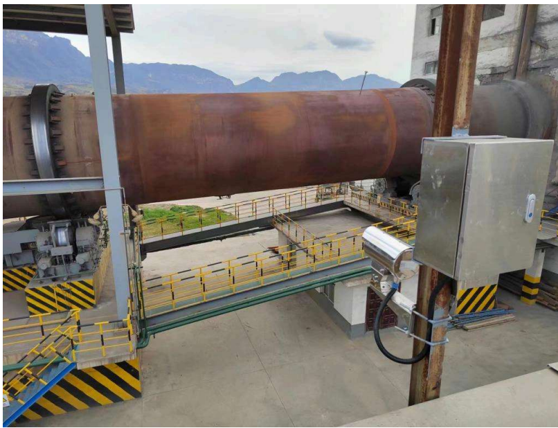
Fig.1. Product and installation diagram of HIRDA-Kiln-K rotary kiln shell infrared thermal imaging online temperature detection and analysis system
